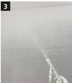
**3** Spray StoSilent Decor M onto the dry StoSilent Top Basic intermediate layer using circular movements. Alternatively use a hopper gun in accordance with the Technical Data Sheet.
