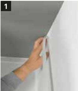
**1** To prevent crack formation, separate off neighbouring surfaces or structures (wall junctions, columns, window or door frames made from metal, timber, etc.) using Sto-Stucco Tape.
