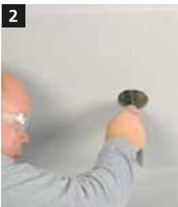
**2** Remove any remnants of the acoustic panel and the adhesive from the opening.
