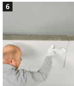
**6** Fix the panels in the bond with an offset of at least 200 mm. They should be flush over the area and tightly butt-joined. Avoid cross joints. Avoid contaminating the visible side of the panel.
