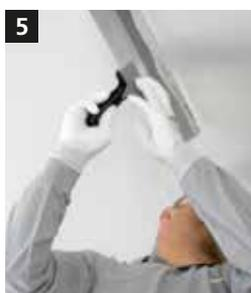
**5** Applying uniform pressure, smooth the material using a wide smoothing trowel, holding it at an angle of approx. 10°. In doing so, trowel off as little material as possible. First smooth the areas along the edge, and then work on the entire surface. Deburr the entire area again afterwards.
