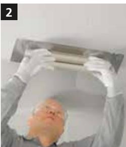
**2** Apply StoSilent Top Basic onto the dry StoSilent Top Basic intermediate layer starting from the corner or the edge. At this stage, the appearance is of secondary importance. It is much more important to apply a sufficient amount of material for the next step.
