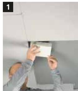
**1** Apply adhesive to the full surface of the StoFix Quader and press approx. 2 mm into the ceiling.
