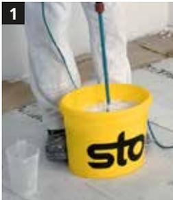
**1** Stir StoSilent Decor M prior to application (if applying by machine, no additional water is necessary).
