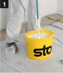
1 Adjust StoColor Climasan to application consistency according to the Technical Data Sheet. Add as little water as possible.
