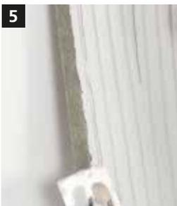
**5** Apply StoSilent Coll MW over the entire rear surface of the panel (full-surface wetting) and tooth with a 10 x 10 mm toothed trowel at an angle of 45°. Then apply an all-around adhesive bead (approx. 5 mm thicker than the combed adhesive).
