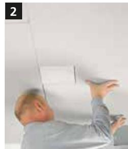
**2** Then bond acoustic panels to the rest of the surface and fill with the joint filling compound StoSilent Filler so that it is smooth.
