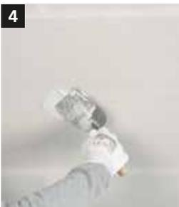
**4** Finally, fill the surface with the joint filling compound StoSilent Filler so that it is smooth.
