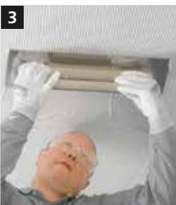
**3** Tooth in a criss-cross pattern using a 4 x 4 mm toothed trowel, whereby the 2nd tooothing runs parallel to the main incidence of light. Press on the toothed trowel strongly and uniformly at an angle of approx. 30°, ideally until you hear scraping on the intermediate coat.
