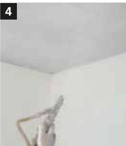
4 After the second spray application and 24 hours of drying time, the StoColor Climasan surface is finished. The substrate is now only slightly visible.
