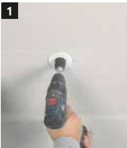
**1** Mark StoFix Zyrillo on the acoustic panel. Then mill the marked area out of the acoustic panel.
