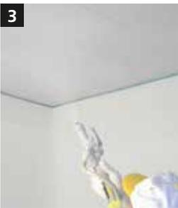
3 Spray StoColor Climasan directly onto the acoustic panels in two to three spray applications using circular movements at a distance of 50 to 70 cm. Observe the drying times between the spray application cycles.
