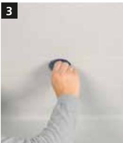
**3** Apply adhesive to the full surface of the StoFix Zyrillo and press approx. 2 mm into the opening.
