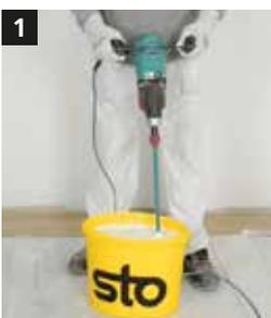
**1** Adjust material to application consistency in accordance with the Technical Data Sheet. Add as little water as possible. For white and tinted StoSilent Top Basic, a smaller quantity of water is required to achieve an optimal application consistency.
