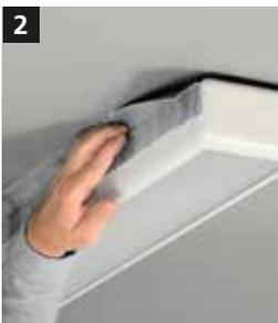
**2** Mask ceiling installations such as lights, speakers, fire alarms, and service hatches with StoSeal Band BK sealing tape so that they are airtight.
