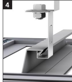
4 Connect StoSilent Modular 100 by hanging its carrier profiles into the connecting hooks and align.
